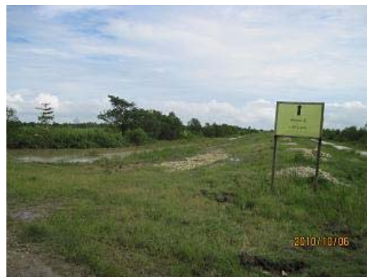
Photo-20: Road No. 5 branches off from Road No.1 near Bogale. Its embankment was completed but not yet paved due to the problem of soft soil.
