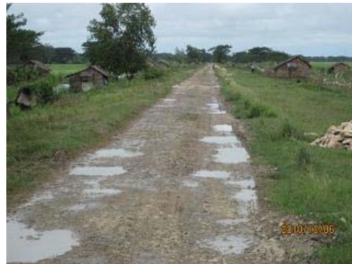
Photo-13: Unpaved roads cannot bear the load of a heavy vehicle, as a result the road surface is easily damaged in a short term of time.
