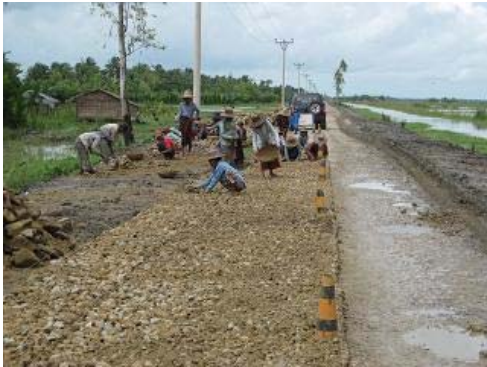
Photo-24: Surface treatment works for road widening.
