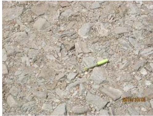
Photo-11: Surface of Metalled road is not very smooth, consequently vehicles can run only at speed of around 20km/h or so.
