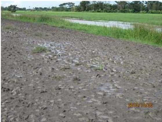
Photo-21: The left photo shows the surface of embankment of Road No.2, which branches off from Road No.1 at Mawlamyinegyun. This section is one of the most problematic sections, where severe settlement occurred. At this point, a settlement of 2 feet during one year was observed. But the embankment of Road No.1, which is located at the same place, is quite stable without any settlement. Therefore, the cause of the settlement does not seem to be the strength of ground, but the quality of soil material for embankment itself. In fact, the material of embankment appears to be "mud" rather than "soil".
