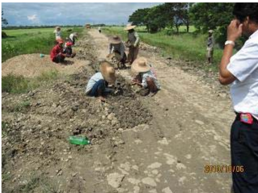
Photo-14: Road Construction Special Unit (RCSU) was maintaining road surfaces.
