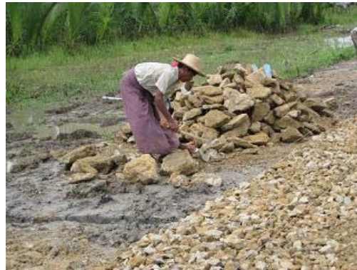
Photo-25: Aggregates were being spread manually. But the Team considered that the strength of “embankment” or “subgrade” should be checked.
