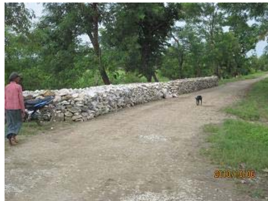
Photo-18: Aggregates for the Matelled surfaces were hauled from a quarry of 80km away of the site.
