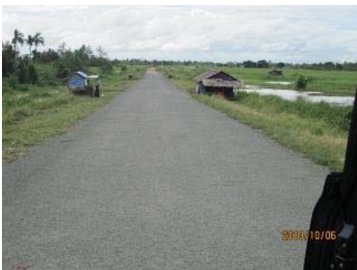
Photo-19: Some sections were paved with bituminous treatment.
