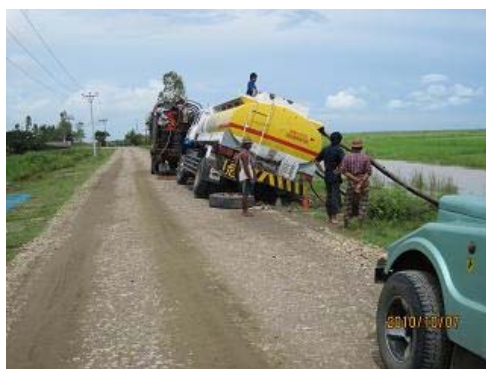
Photo-27: Tires of a lorry were buried into the newly constructed portion of the embankment.
